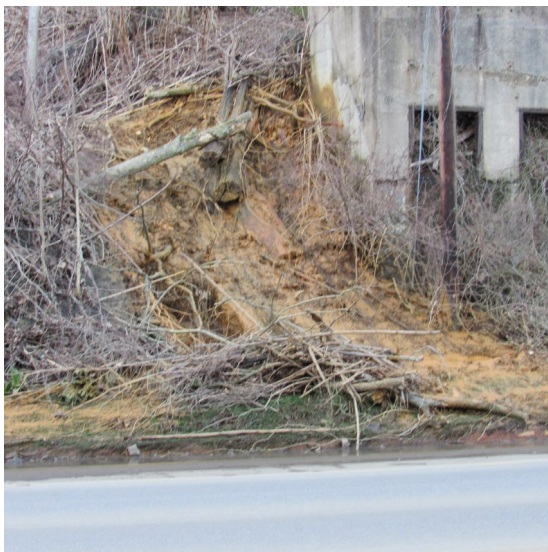
The source location along Franklin Street in suburban Johnstown that produced a surge of AMD contaminated water, near and into the Stonycreek River.
