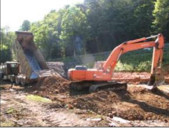
Soil from the Route 219 Construction Project is delivered and spread during construction of the Rock Tunnel Rehabilitation Project. *Photo by Len Lichvar*
